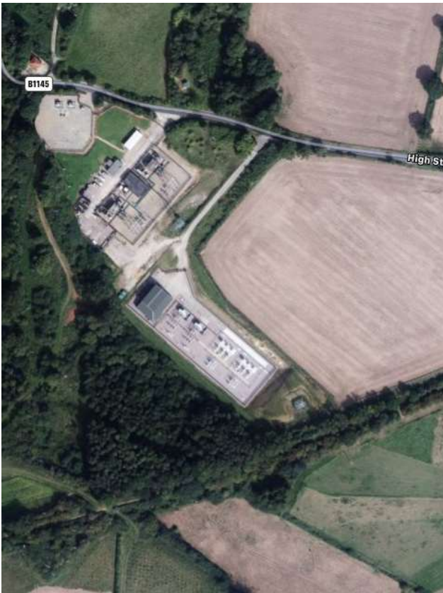
Sheringham Shoal substation
